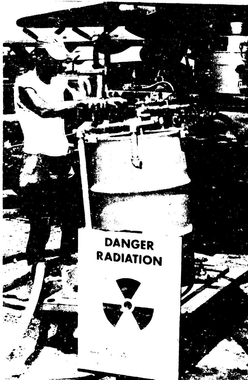
Figure 5.8 Operator adjusting control valves on the hot-liquid-jet unit. The unit is secured on top of the barrel which holds the detergent solution.
